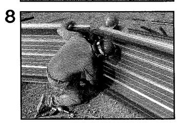
ROOF PANELS ARE INSTALLED IN A VERTICAL POSITION SOUARELY ON THE FLAT LEG OF THE 90 DEG. CORNER
