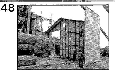
SPREADER BEAM IS NOT REQUIRED. USE TWO POINT PICK AT RIDGE.
