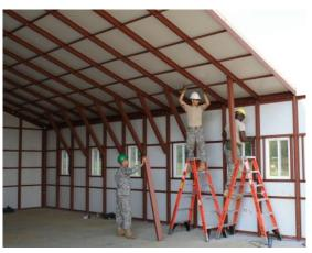
Knee and ridge braces are installed as wall and roof panel sections are set in place.
