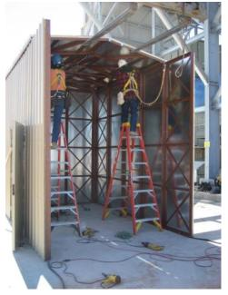
Roof panels are hinged at the ridge. The roof structure is completed with roof trusses comprised of a tension tie and web braces that bolt to the roof panel in the air.
