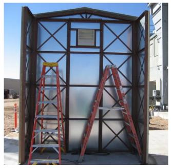
Additional panels create the first complete endwall. A gable closure panel with factory attached trim creates the start of the gable roof shape.
