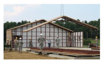
6' roof sections are assembled on the ground and lifted into place by the crane.
