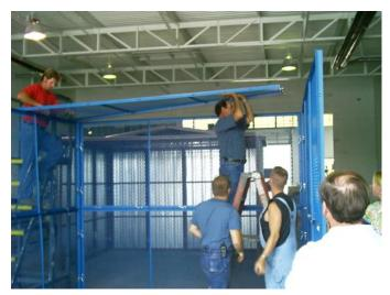
Roof Panels Placed onto Wall Panels
